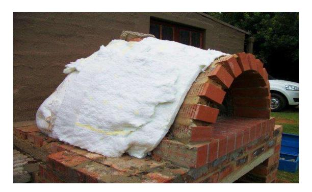
15. Start closing the oven by building and outer skin with clay bricks.
