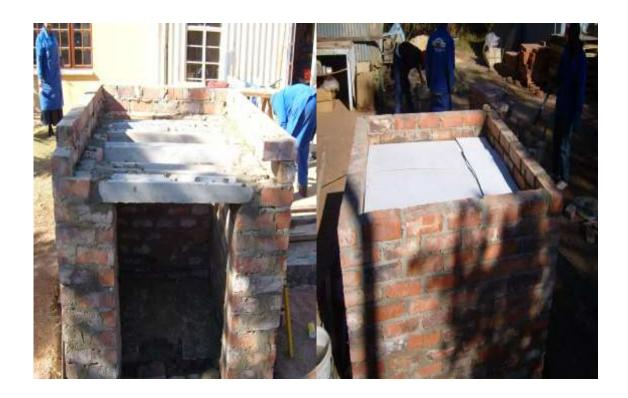
4. Construct this base with a solid concrete slab, 1m high from finished floor level.
