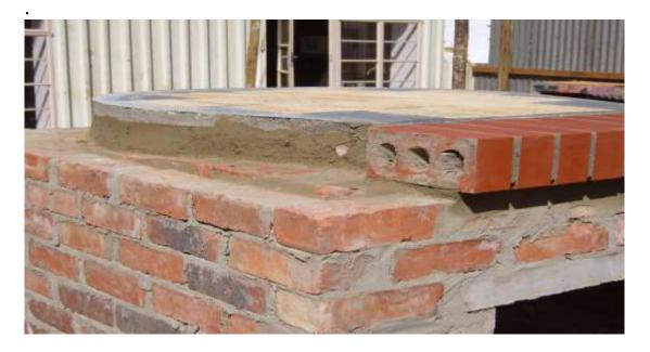
8. Install the brick sill in front of the oven, with the top of the sill level with that of the pizza ovens floor.
