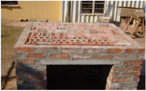
6. Make a dry mix topping with sand and cement. This goes on top of the clay bricks 70mm thick. (Compact it a little). It is important that the topping is completely level to support the floor of the oven.
