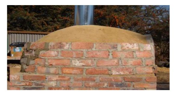
16. Continue by plastering the oven, and cork the brick arch's gaps that it can blend in with the plaster.
