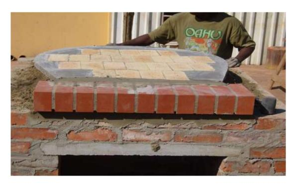
9. Proceed in placing the dome on top of the floor
